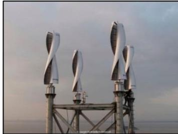
Fig. 8 Four Windside WS-4B wind turbines producing power for a radar station in China, (courtesy of Windside Production Ltd 2009)
