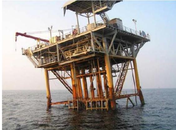
Fig. 1 Platform with suspected foundation failure (Aggarwal *et al.* 1996, Ishwarya *et al.* 2016)
