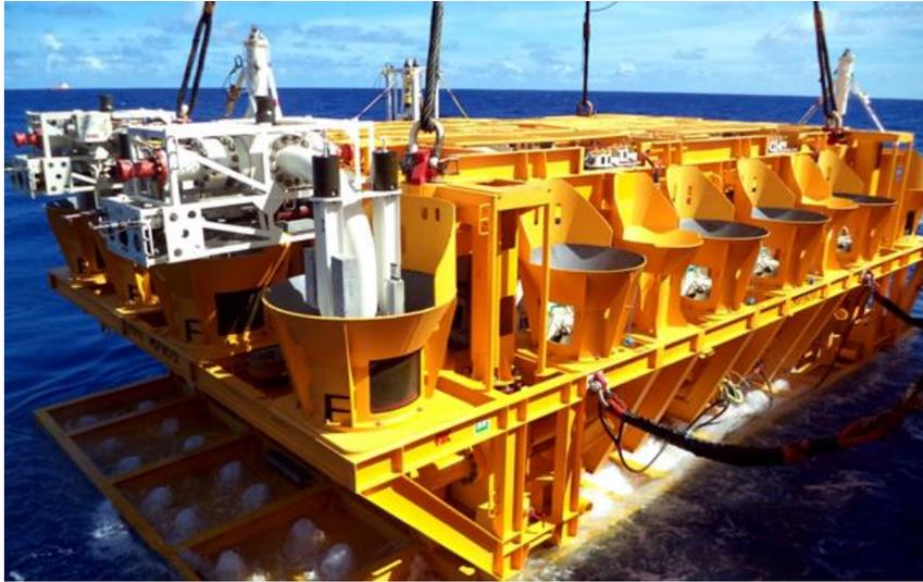
Fig. 1 Subsea manifold crossing the splash zone, courtesy from Petrobras
