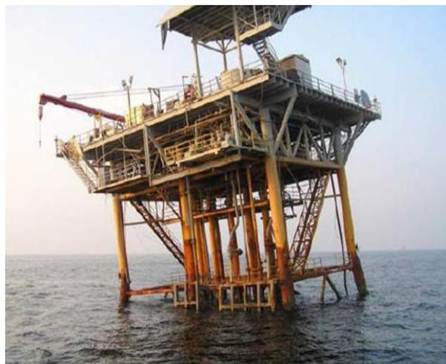
Fig. 1 Platform with suspected foundation failure (Aggarwal *et al.* 1996, Ishwarya *et al.* 2016)
