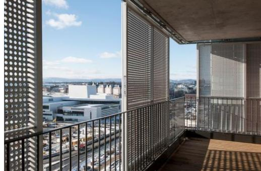
Fig. 5 Example of fixed shading device
