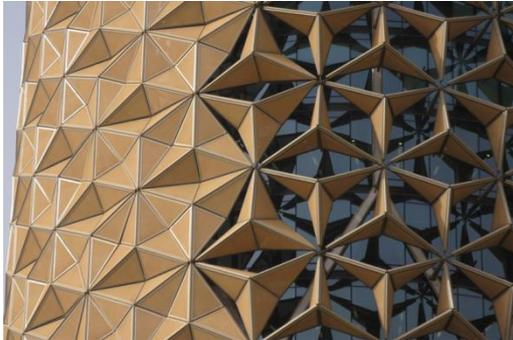
Fig. 4 Example of kinetic shading device
